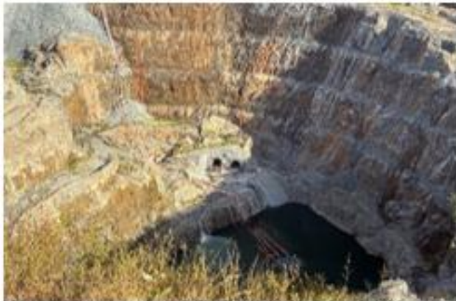
Tailrace tunnels are visible at the bottom of the Eldridge Pit
