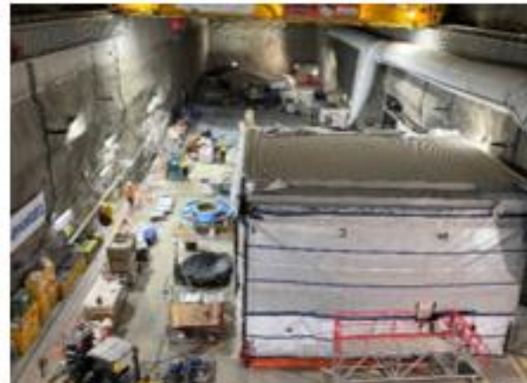
Powerhouse fit out underway - 250m underground
