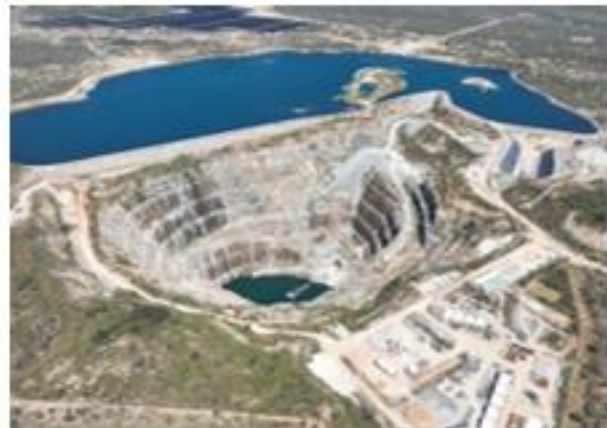
Aerial of Wises Dam (upper reservoir) and Eldridge Pit
