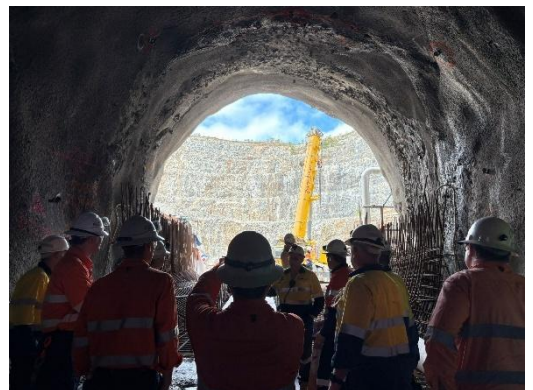
The Board inside the one of the tail race tunnels looking out into Eldridge Pit
