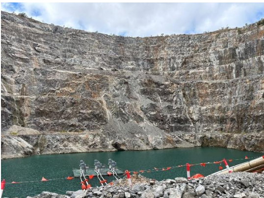
Eldridge Pit is the lower reservoir and will receive the water from the upper reservoir (Wises Dam) after it passed through turbines.
