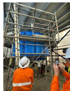
The Board inspecting unit 1 stator assembly
