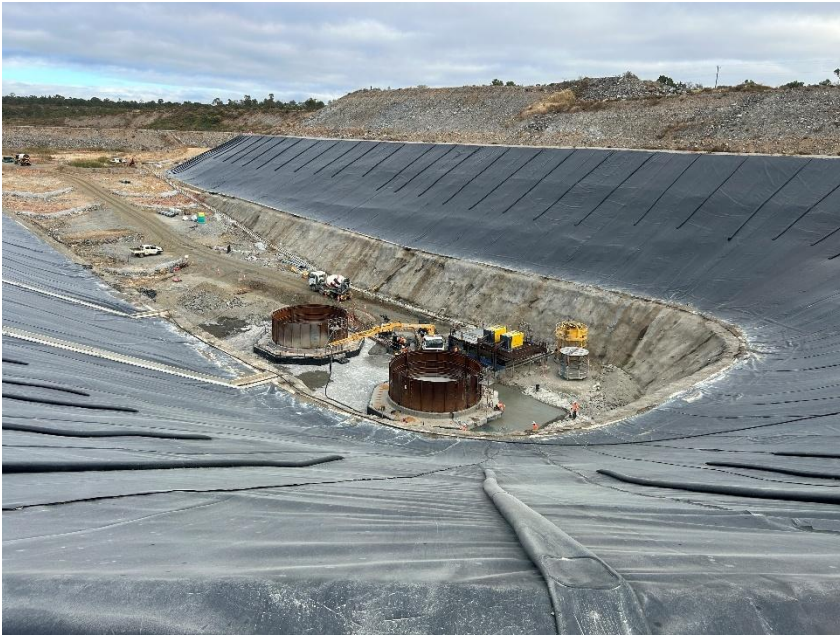
Closeup of the Intake Canal and the two Intake Shafts.
